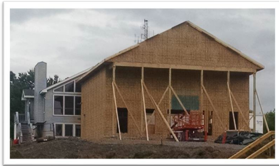
Courthouse Renovation and Expansion to Existing Courthouse (Before)
