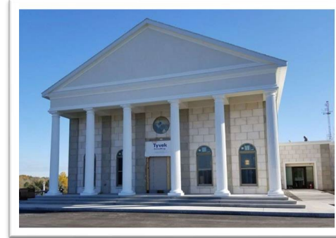
Courthouse Renovation and Expansion to Existing Courthouse (After)
