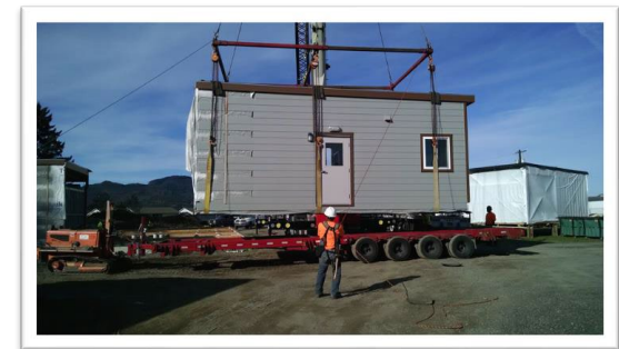
Transporting Modular Unit
