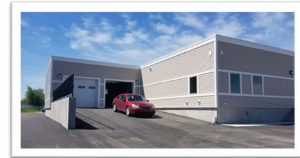
Sally Port for Tribal Court
